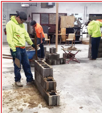
Apprentice Bricklayers Brennan Jennewein, Sean O'Neill & Spencer Newton are shown building block leads during a recent Level 2 Apprentice Training Class.
